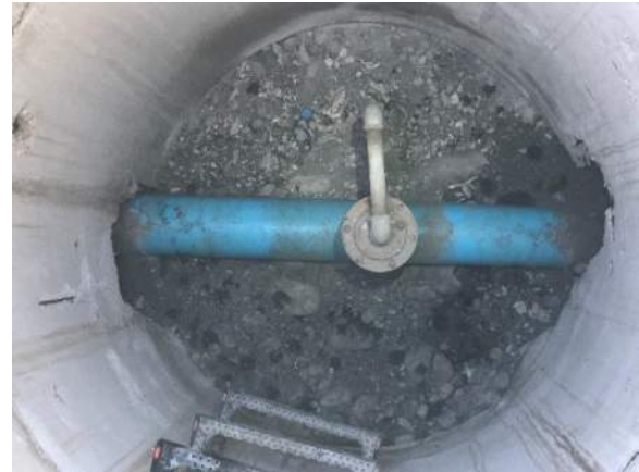
FIGURE 4 – AIR/VACUUM RELEASE VALVE VAULT INTERIOR
