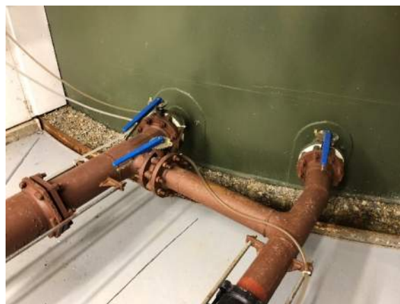
FIGURE 6 – ADJACENT TANK ENTRY AND EXIT PIPES
